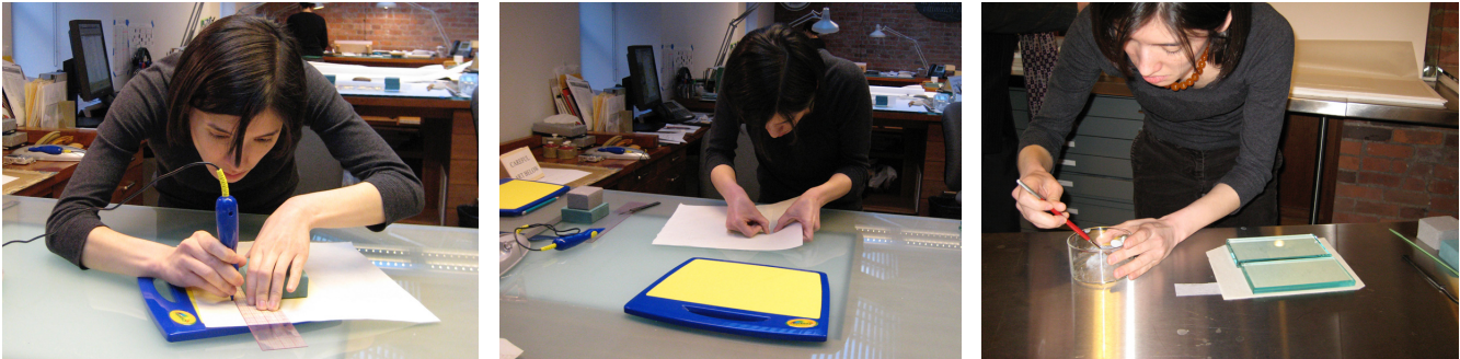
ABOVE, LEFT TO RIGHT Fig. 2. Following the traced line with the Crayola Cutter to create a perforated outline of the drawing Fig. 3. Pulling the perforated line apart to release the inlay Fig. 4. Pasting up the edge of the drawing with wheat starch paste before attaching it to the inlay LEFT Fig. 5. The drawing adhered to the inlay
